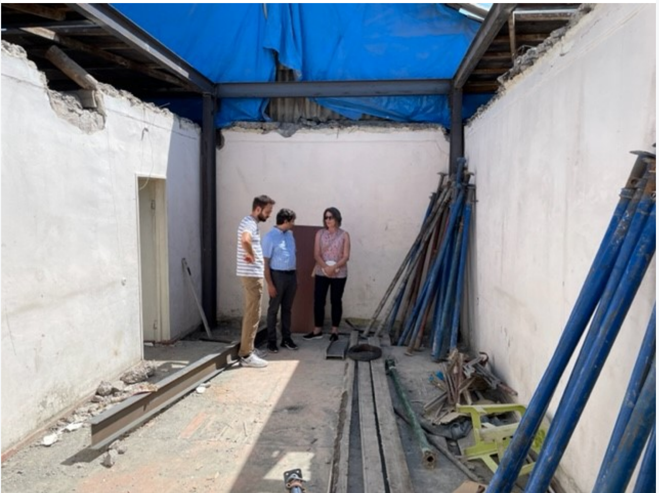
Second floor being added
